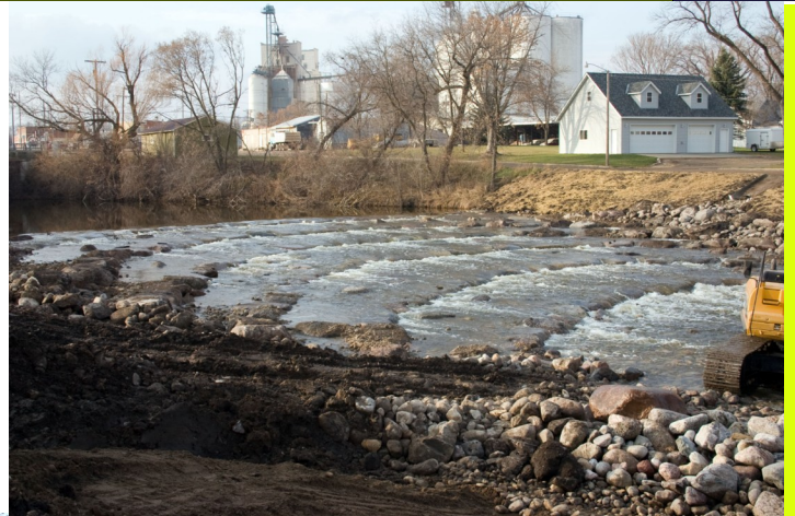
A rock-weir rapids just upstream of the old dam site in Dawson along the Lac Qui Parle river.
